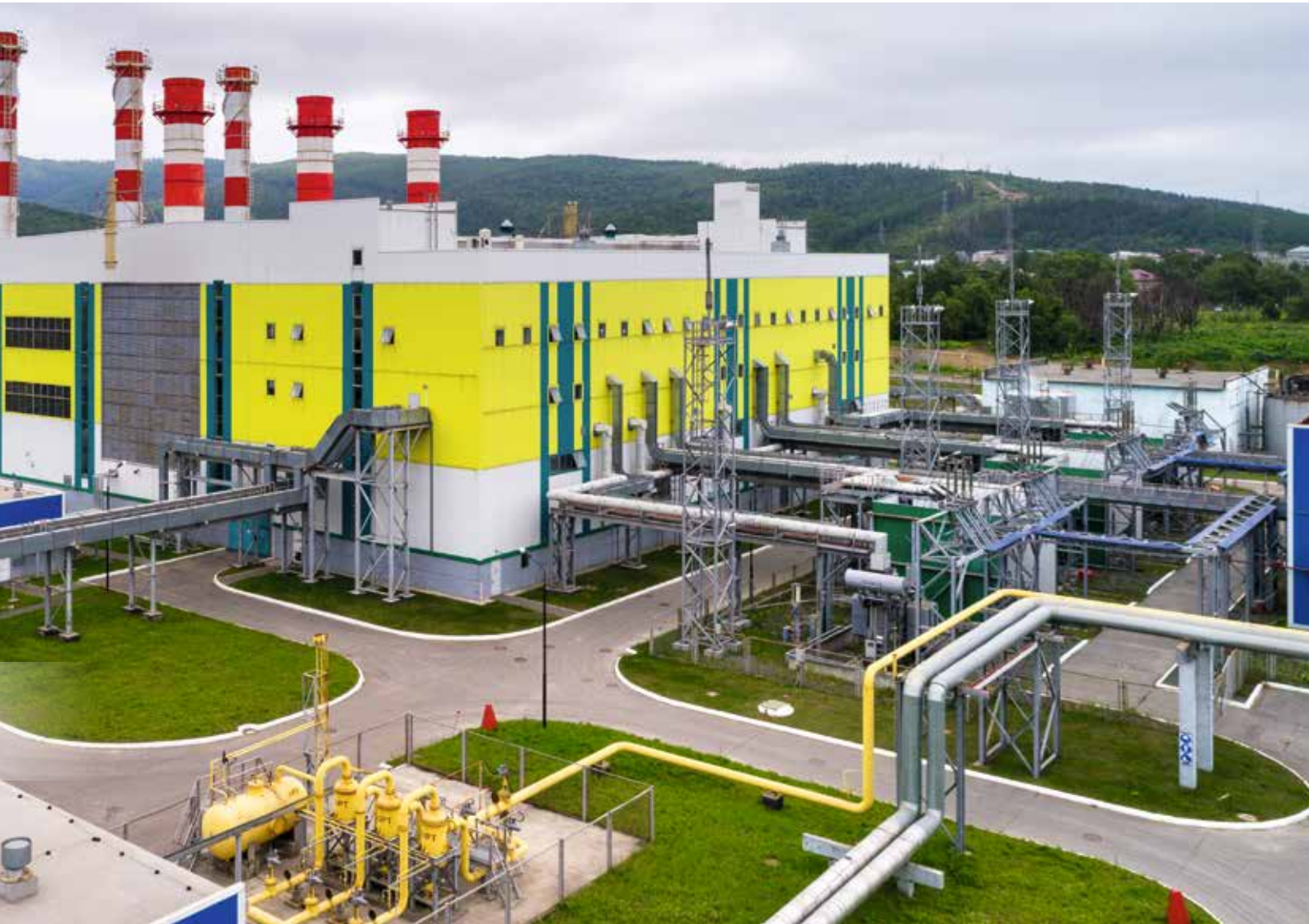
Yuzhno-Sakhalinskaya CHPP-1, unit No. 4
